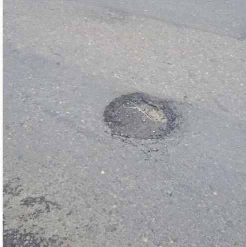
Gambar 2.20 Lubang (*potholes*)
