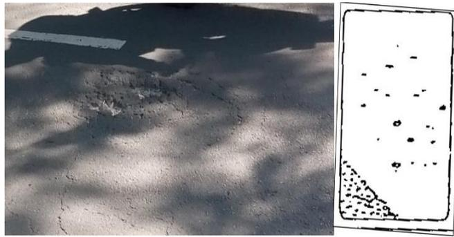
Gambar **Error! No text of specified style in document.**21 Pelepasan Butir (*Raveling*)
