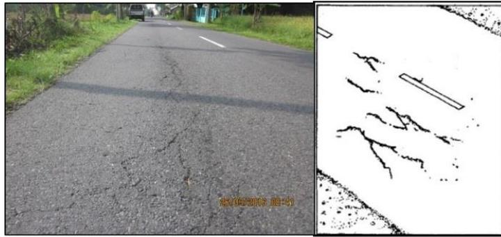
Gambar **Error! No text of specified style in document.** 6 Retak Halus (*Hair Cracks*)
