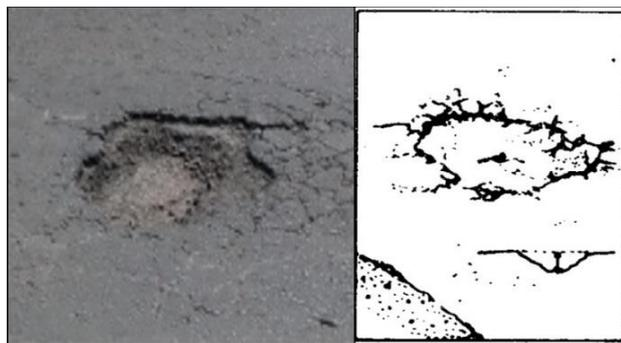
Gambar **Error! No text of specified style in document.**20 Lubang (*Potholes*)
