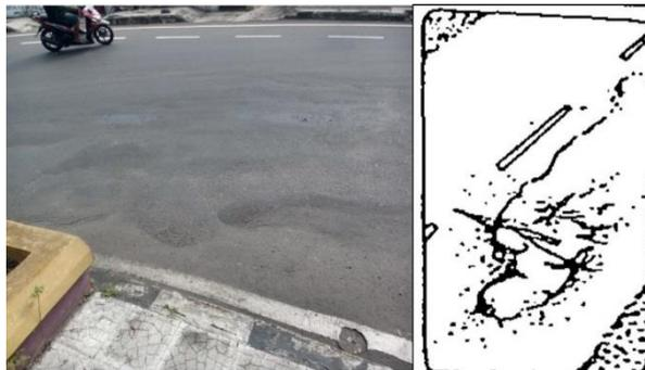
Gambar **Error! No text of specified style in document.**..24 Kegemukan (*Bleeding Or Flushing*)
