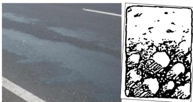
Gambar 2.19 Pengausan (*Polished Agregat*)
