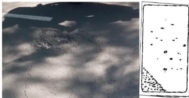
Gambar 2.31 Pelepasan Butir (*Raveling and Weathering*)
